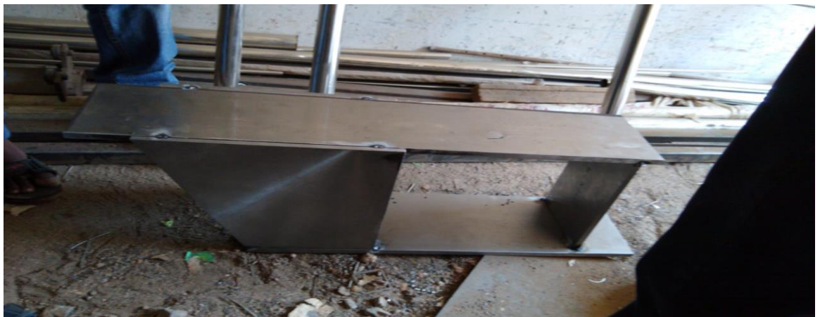
Figure 4.1: Fabrication of Base.
